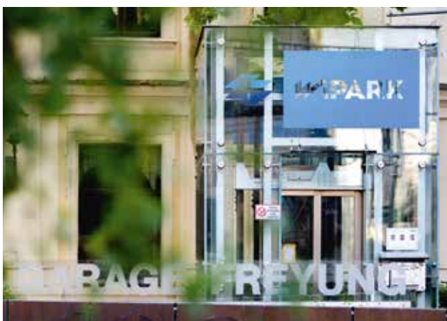
Safety at WIPARK car parks and the ease with which users can navigate the facilities are regularly assessed.
