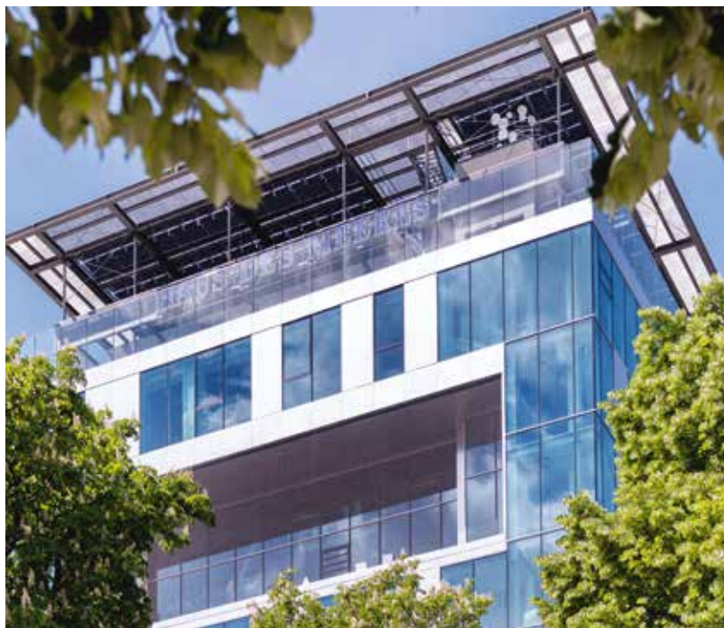
The new solar array on the roof of the Haus des Meeres - Aqua Terra Zoo comprises 202 special bifacial glass/glass photovoltaic modules to generate electricity from below as well as above.
