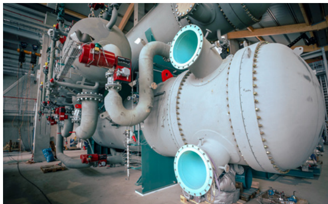
Wiener Stadtwerke is producing climate-neutral district heating with one of the most powerful large-scale heat pumps in Europe , which is being built on the site of the ebswien sewage plant in Simmering.
